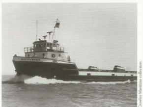
The  $165 \times 36 \times 15$ -ft. supply boat Rig Pusher was added to the fleet in 1967 for use in supporting offshore drilling and construction activities.
