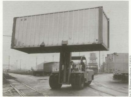
Containers were loaded by forklift and crane onto PSAVL barges.
