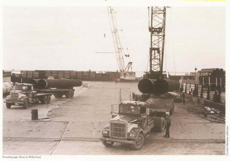
size, it was the largest sealift in the project's history, with forty-seven barges amassed to carry 160,000 tons of cargo. That included 179 modules reaching as tall as nine stories and weighing up to 1300 tons each, and 40,000 tons of general cargo—virtually everything necessary to sustain North Slope pipeline construction over the following twelve months.
