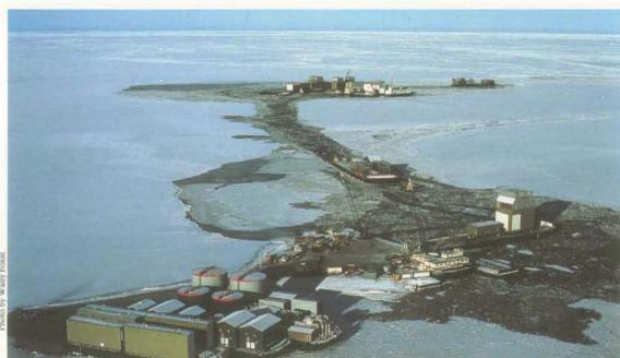
Oceangoing module barges wait together offshore as three tugs maneuver one barge at a time, lightering modules to the dock.
