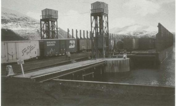
Railcar transfer bridges in Whittier (shown) and Seattle allow for easy roll-on/roll-off loading and offloading of railcars.
