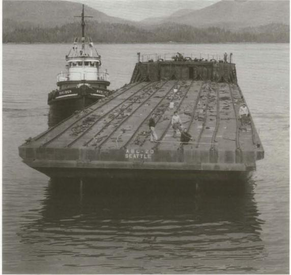
Barge ABC 20, operated by Alaska-British Columbia Transportation Company, was equipped with rails to transport railcars between Ketchikan, Alaska, and Prince Rupert, British Columbia, Canada.
