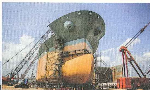
Above and left, the 330,000-bbl barge 750-1 at VT Halter Marine, in Pascagoula, Miss. The ship-like barge has a flared bow rising from a bulbous nose.
