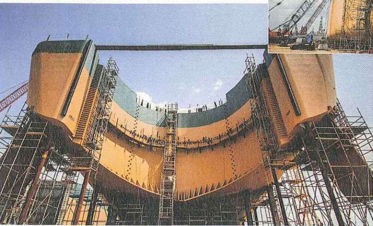
Above and left, the 330,000-bbl barge 750-1 at VT Halter Marine, in Pascagoula, Miss. The ship-like barge has a flared bow rising from a bulbous nose.
