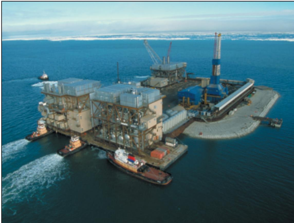
*Crowley's 2001 summer sealift culminated with the delivery of production modules to Northstar Island near Prudhoe Bay. Measuring more than 10 stories high and weighing more than 3,500 tons each, they were the largest modules ever made in Alaska.*
