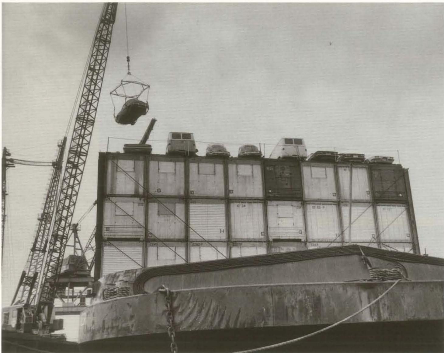
*A crane positions a car on top of a three-high load of containers aboard the barge Whittier. Crowley developed a framework to secure containers for the ocean haul without the need for lashing.*
