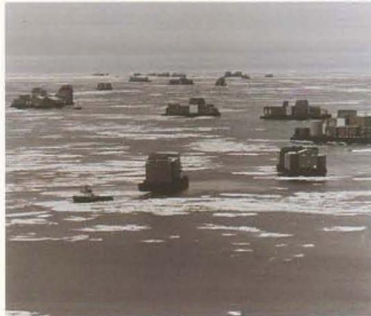
*The 9,000-h.p. tug Warrior tows a 400 x 100-ft. barge loaded with a drilling rig broken down into modular components, 1991.*
