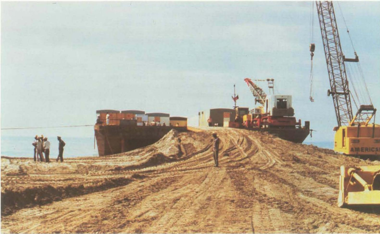
*At a remote beach in Haiti in 1978, Crowley constructed sand ramps to discharge barges loaded with construction equipment and housing.*
